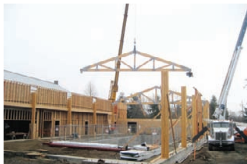
Each truss weighs 6000 pounds.
