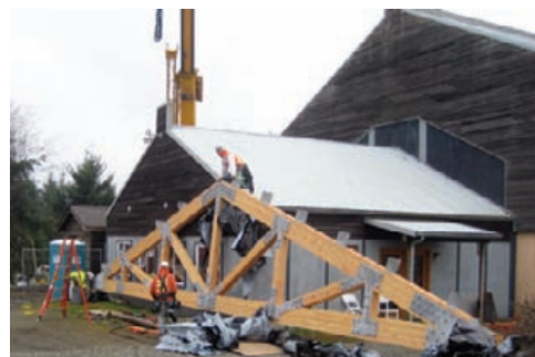
A truss being prepared behind the Mary Johns Room
