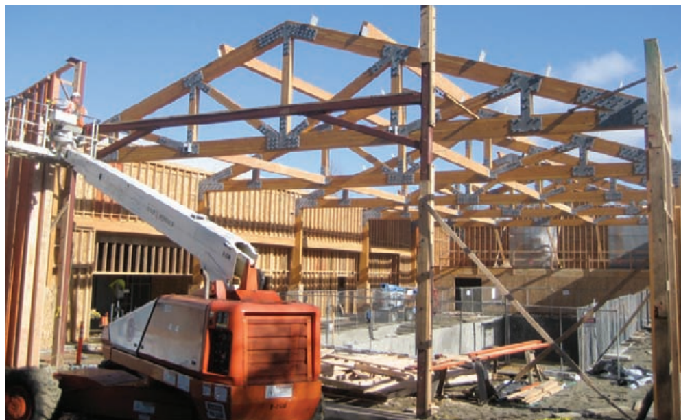
There are 5 trusses and 84 purlins. The purlins are 6" by 16" and 24 feet long. The resulting structure is very strong.
