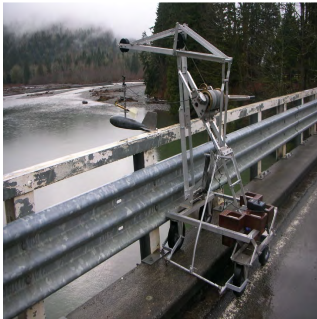
Figure 2 Bridge crane equipped with a USGS Type B reel. (Photo by Washington Dept. of Ecology)
