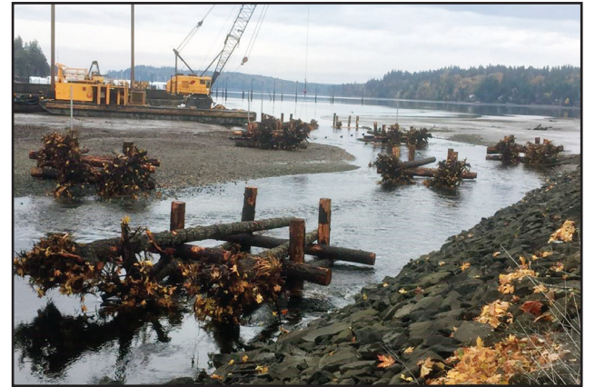
Logjams constructed along Goldsborough Creek, in addition to several other habitat projects, have led to historic runs of juvenile coho.
