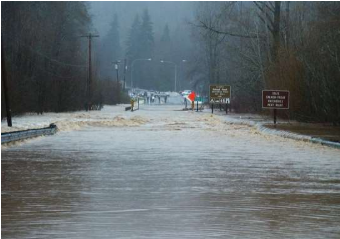
Figure 9-12 U.S. Route 101 North of Shelton - December 3, 2007 Severe Storm Event
